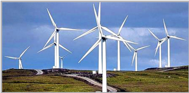
Top to bottom: Power Transmission: Yas Island Infrastructure and Utilities Works Sections, Abu Dhabi. Renewable Power Generation: Onshore Wind Farm, Romania.
